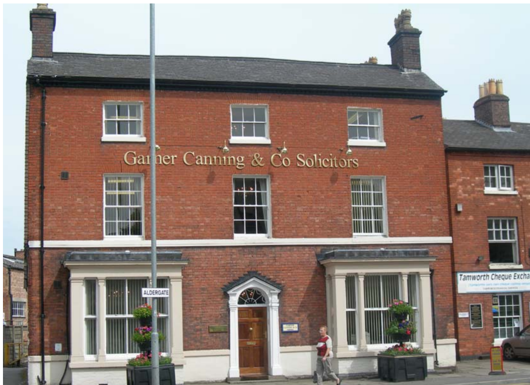
The listed No. 11 Aldergate
