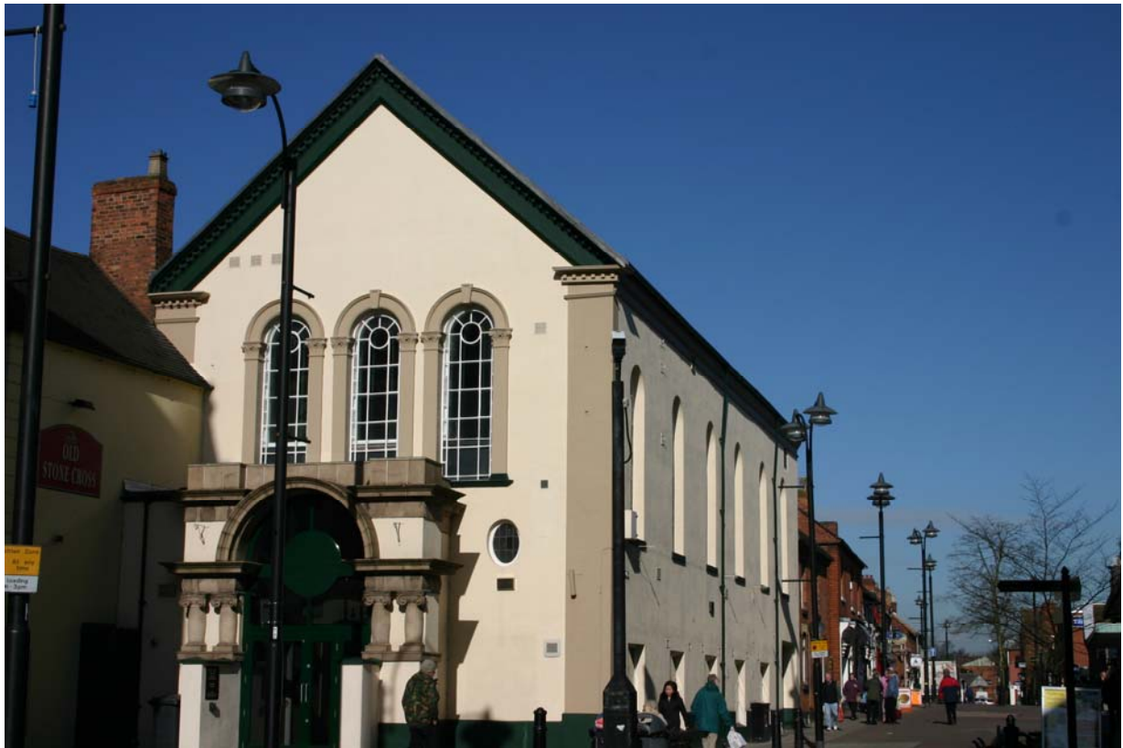
The listed Tamworth Arts Centre, a striking building in a prominent position facing down Colehill
