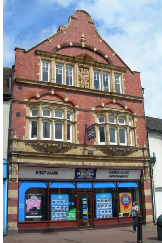
The listed landmark building, No. 37 George Street
