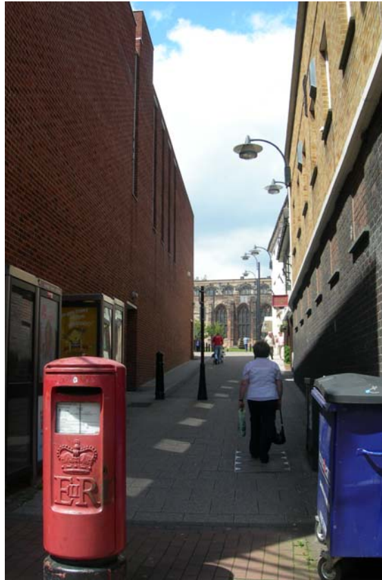
The significant view north to St. Editha's Church along College Lane suffers from late 20th-century redevelopment and clutter
