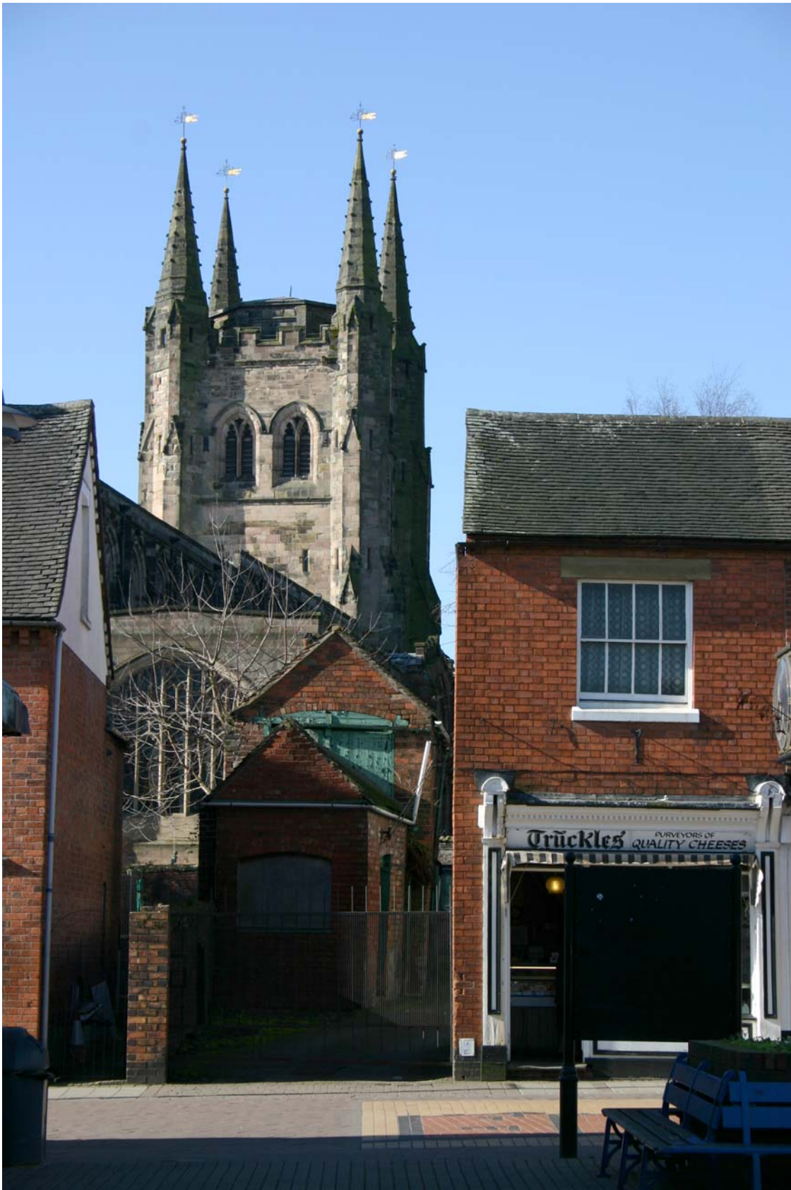
Attractive and significant view through gap in the street frontage to St. Edith's Church, with historic outbuildings in foreground
