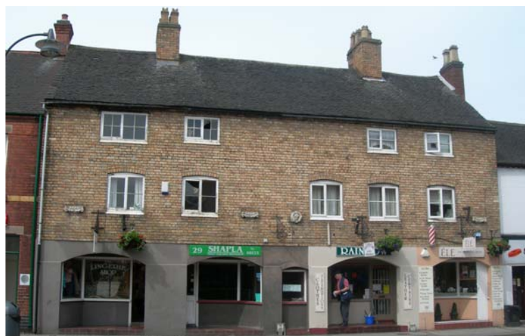
Nos. 27-33 Lower Gungate, also recommended for local listing
