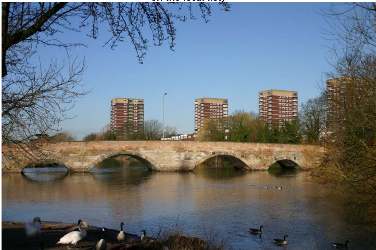
View of Lady Bridge with tower-blocks behind
