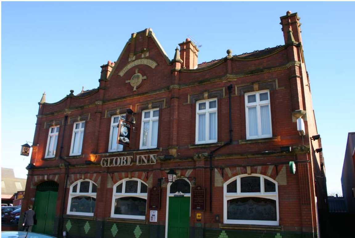
The locally listed Globe Inn, a somewhat isolated but important survivor on the northern part of Lower Gungate
