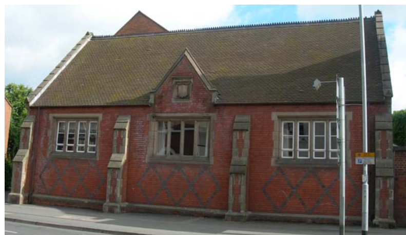
The attractive listed former Peel School on the north side of Lichfield Street
