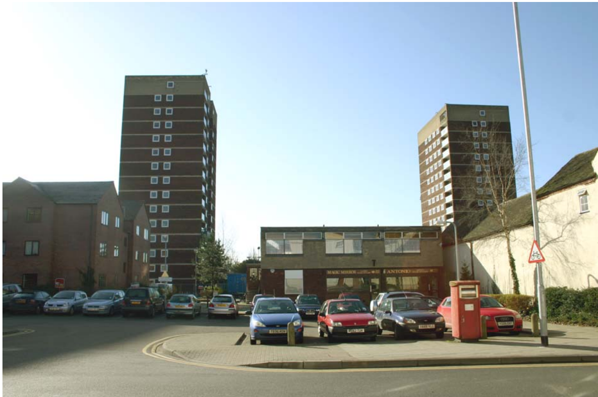
View into the 1960s housing development, with car park creating a rather bleak gap in the streetscape
