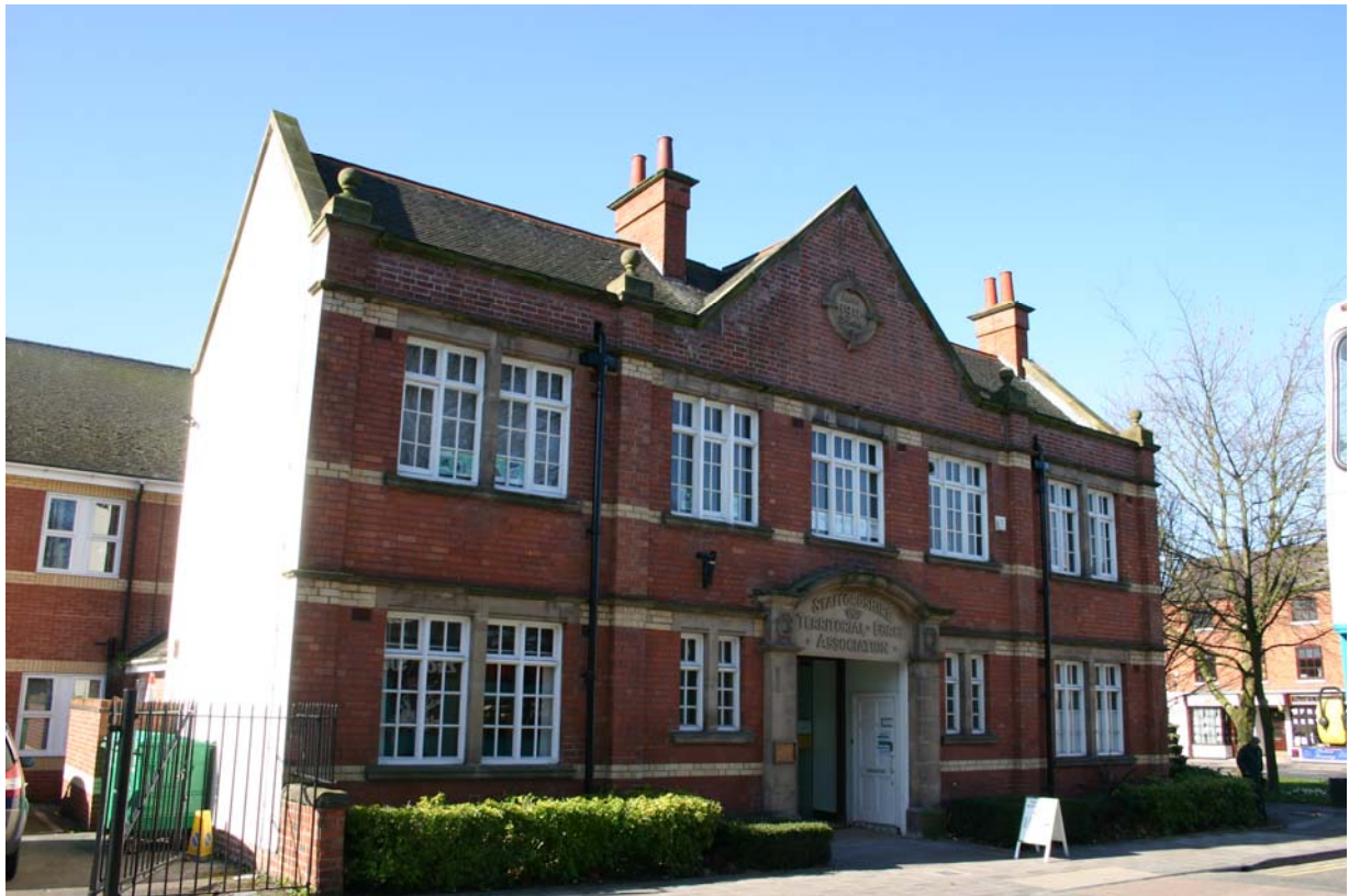
The locally listed former Drill Hall (Philip Dix Centre) with modern extension behind
