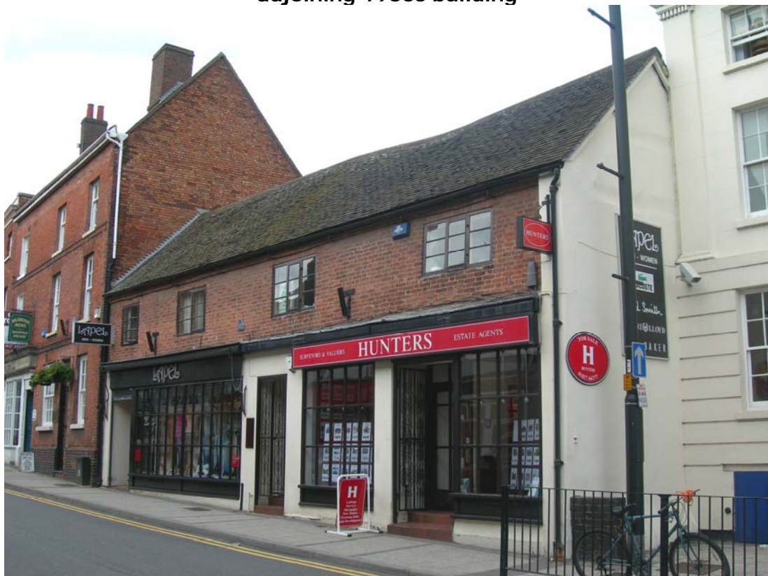
Behind the prominent shop fronts on the listed Nos. 5-9 Bolebridge Street are 17 th -century buildings with timber-framed cores
