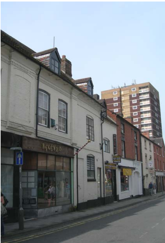
The listed Nos. 66-71, an attractive group on the south side of Church Street
