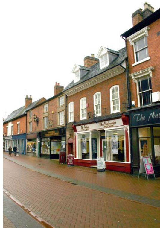
South side of Market Street
