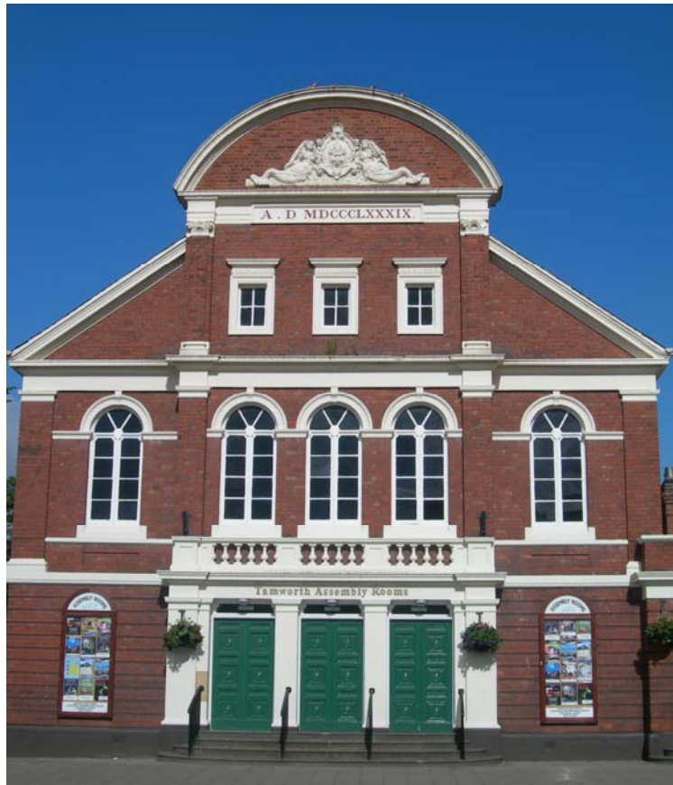
The eye-catching Assembly Rooms
