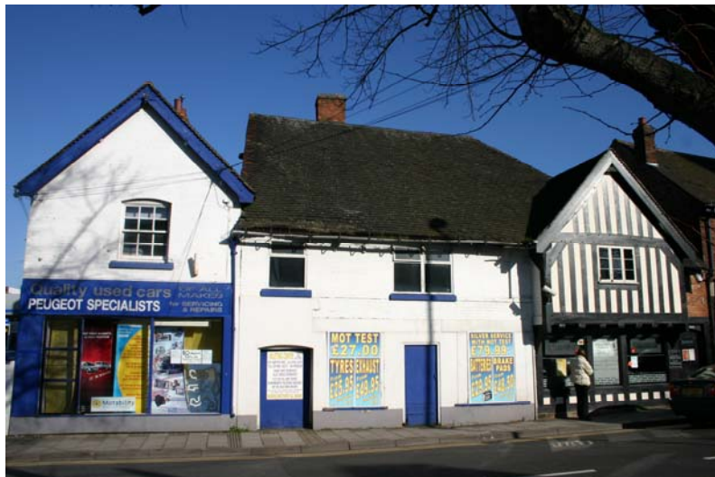
Nos. 110-111, a timber-framed late 16 th -century listed building on the north side of Lichfield Street
