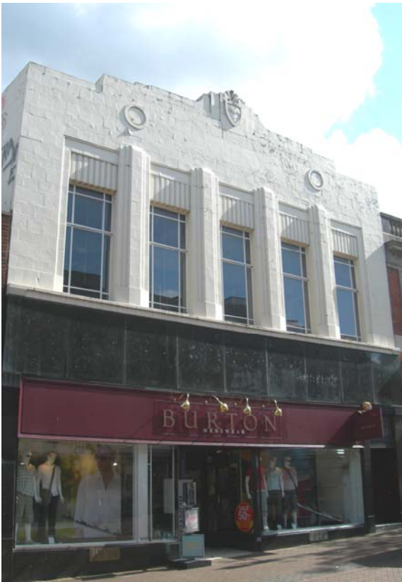
The locally listed Nos. 15-16 George Street: a purpose-built Burton's store, prominent in the streetscape
