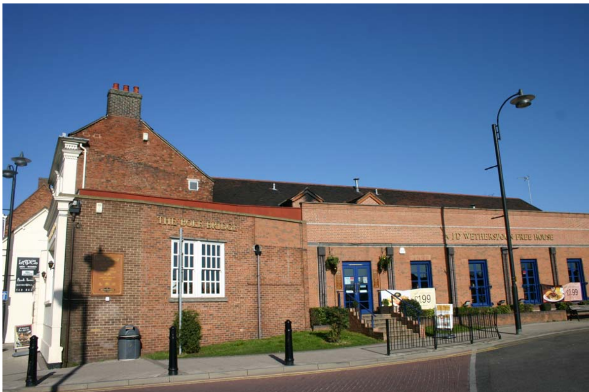
The Bole Bridge public house, with unattractive 20 th -century addition obscuring the earlier rear range
