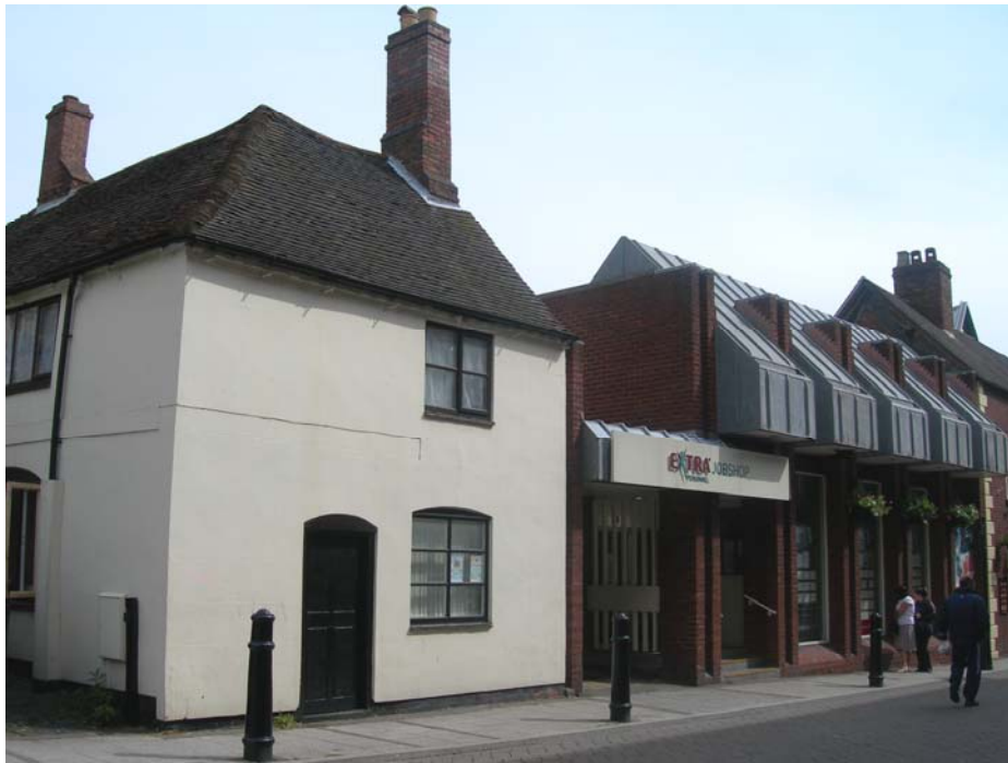
The locally listed No. 29 Church Street adjoining the unattractive No. 31
