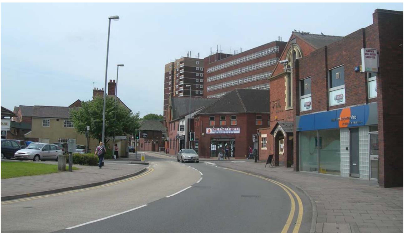
High-rise block and Marmion House rear up behind the smaller-scale buildings on the west side of Aldergate. Also showing the unfortunate design of the late 20 th -century buildings between the Victorian Methodist Chapel and former Congregational Chapel
