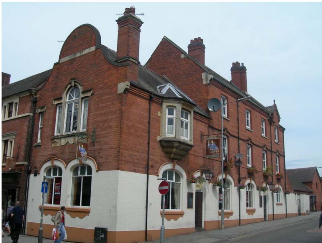
The locally listed Tavern Inn, an attractive building in a prominent corner location, recommended for addition to the local list
