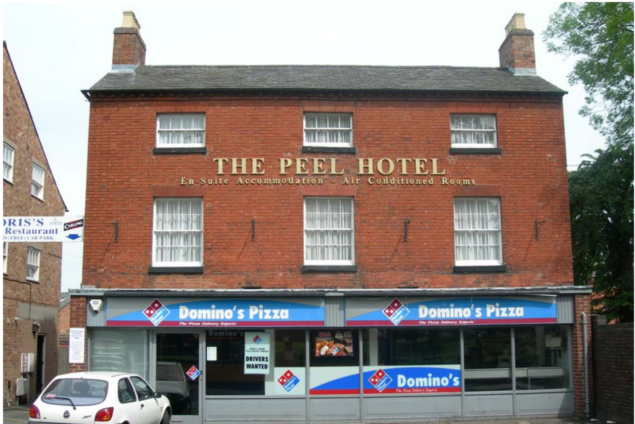
The listed No. 14 Aldergate, unfortunately marred by a wholly inappropriate modern shop front
