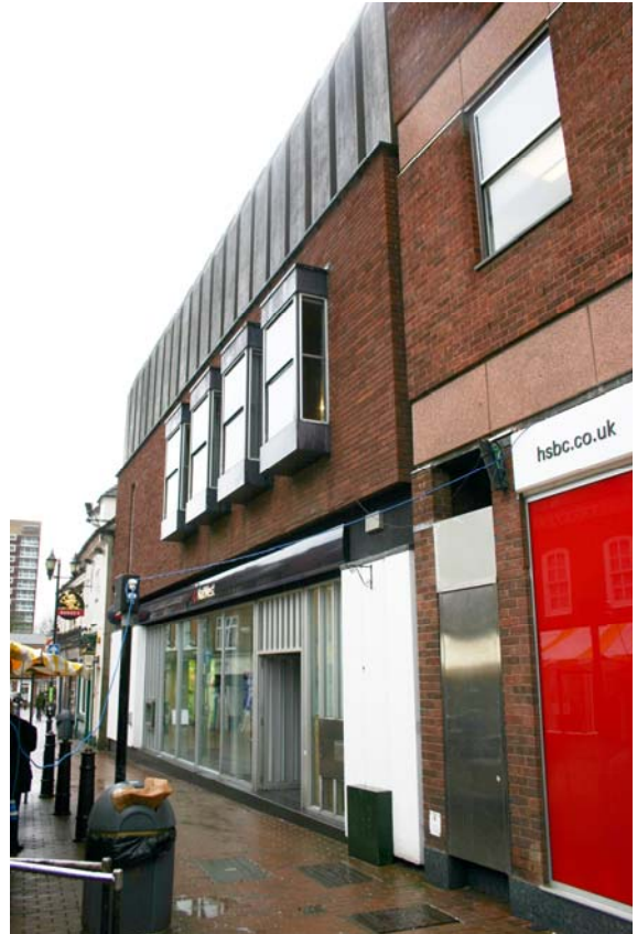
Unsympathetic 1960s buildings on north side of Market Street (NatWest and HSBC)
