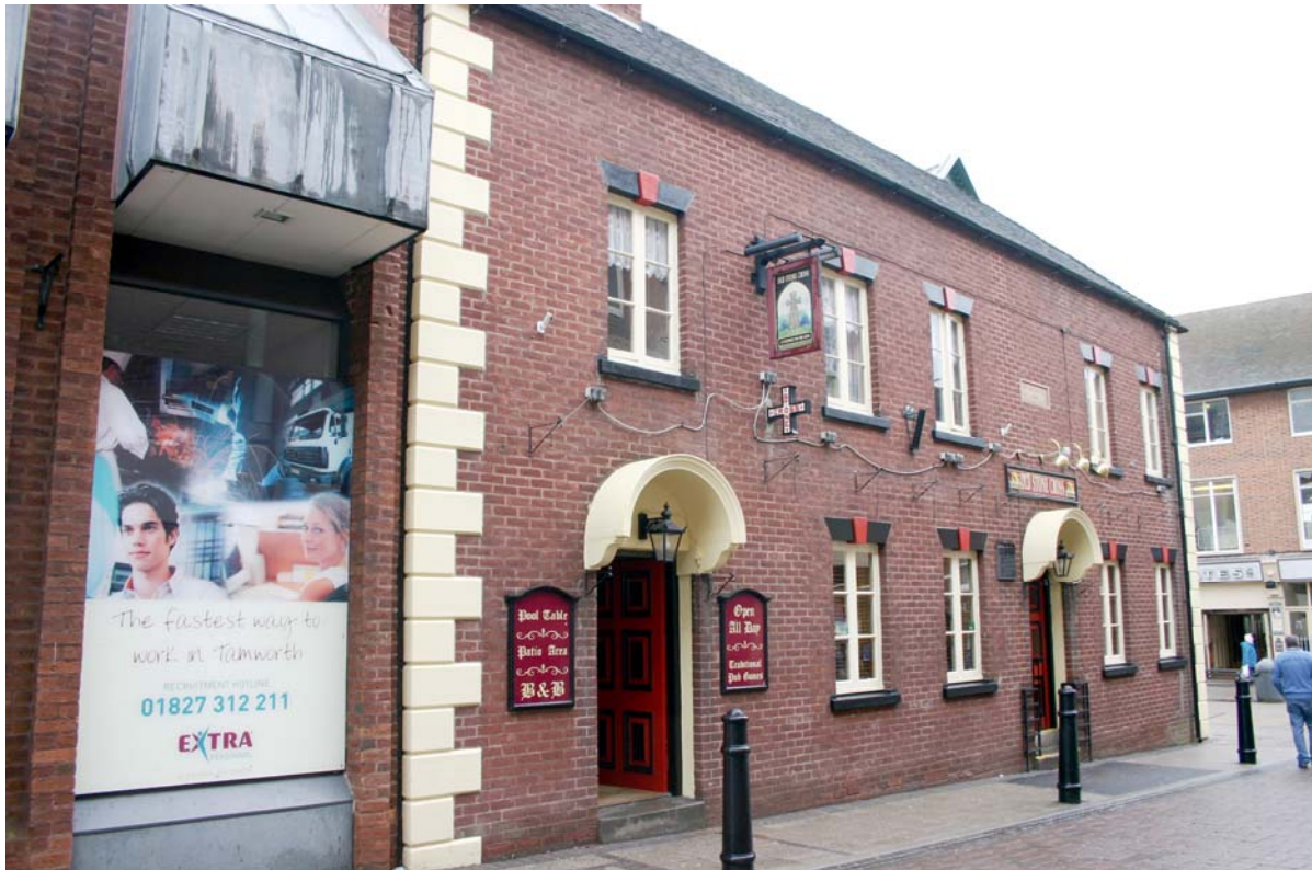
The listed Old Stone Cross public house with reconstructed façade
