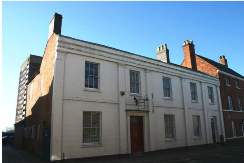
The listed No. 28, also in need of maintenance, stands out for its classical detailing
