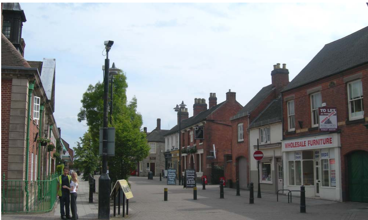
The view south along Lower Gungate demonstrates a better retention of historic character
