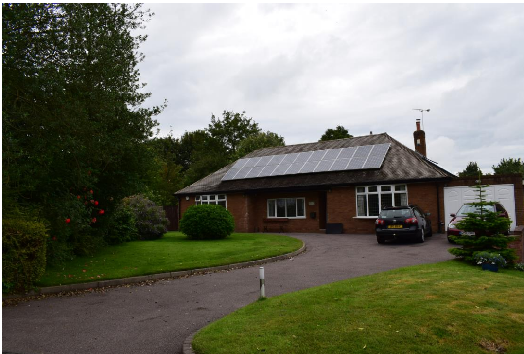
Figure 2: Solar Panels installed along the Amington Old Hall Drive
