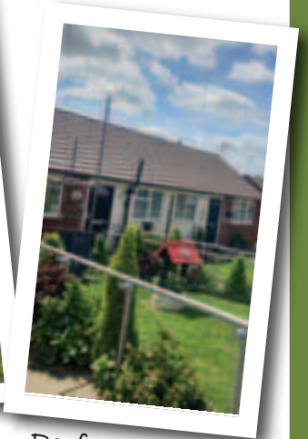
Roofs at Edward Court (After)
