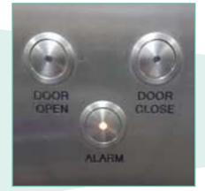
If there is no "Tunstall" button press the button with the word "alarm" beneath it. Hold this button for a minimum of 3 seconds.
